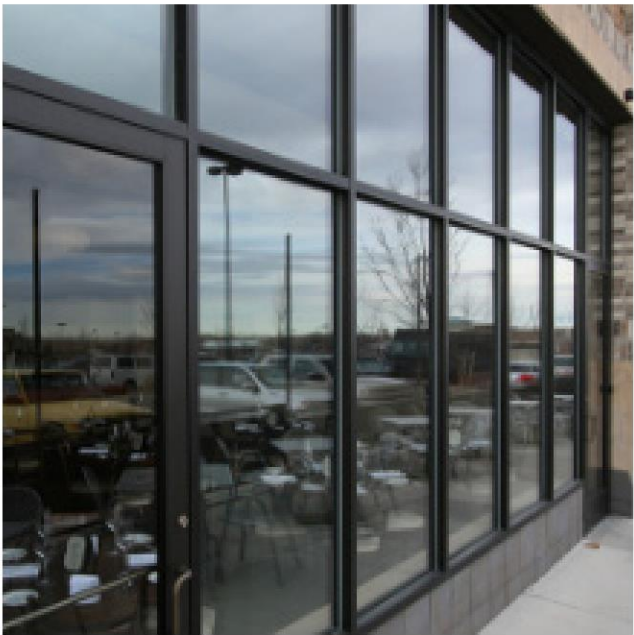
Dark Bronze Aluminum Storefront and Window Systems with Clear Glass (Typ.)
